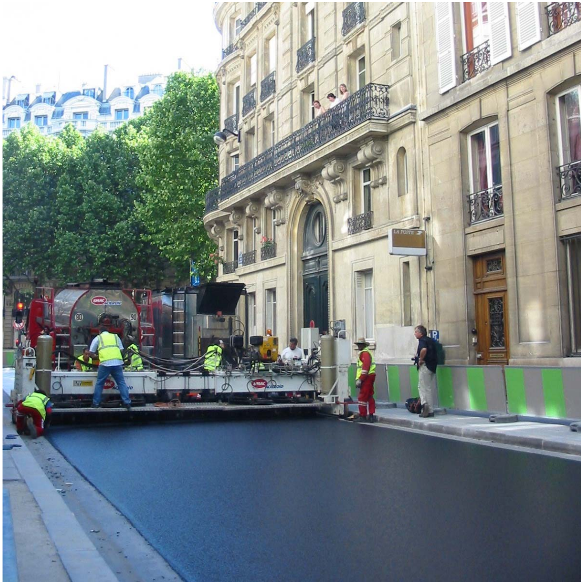
Machine laid mastic asphalt pavement.
