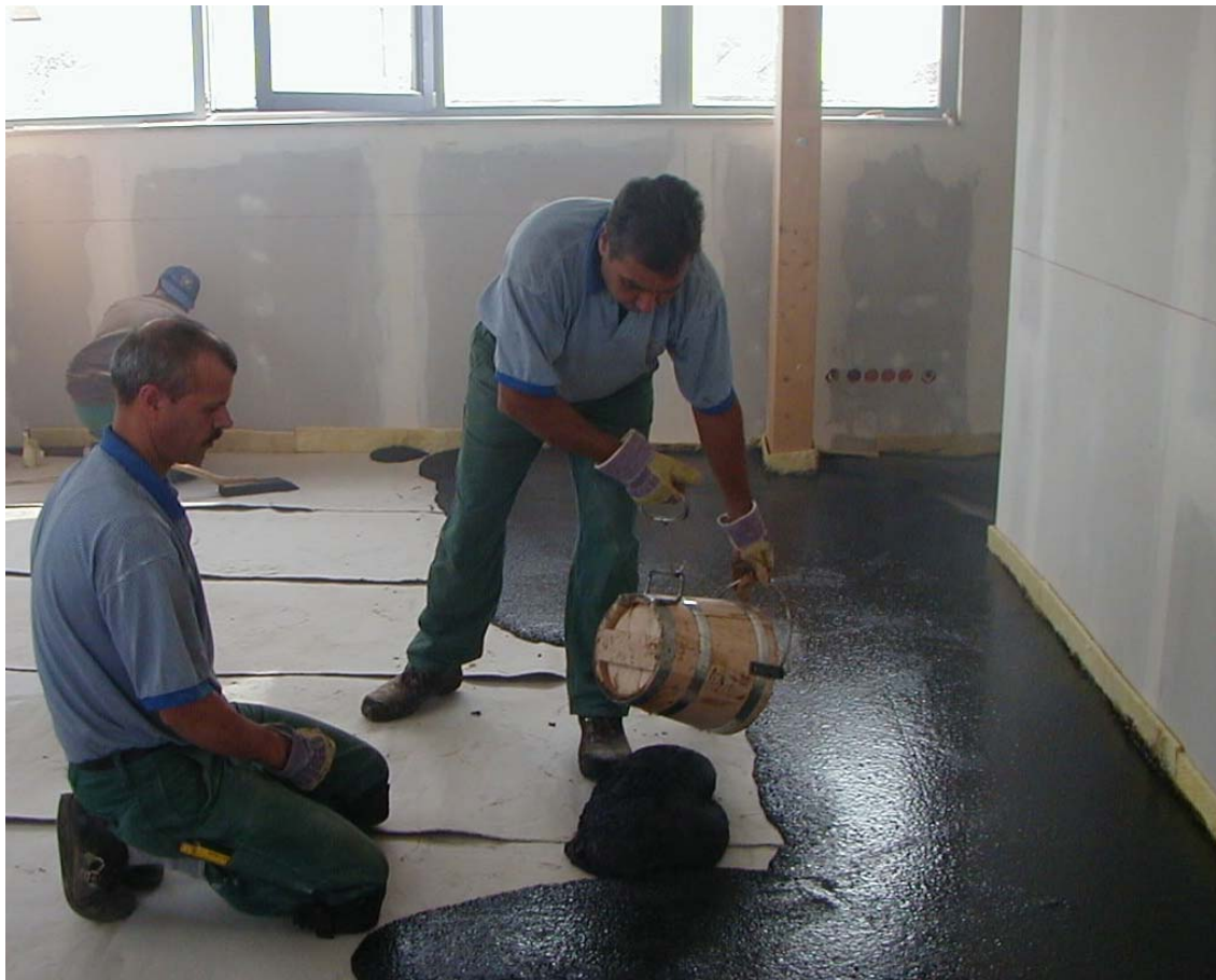
Hand laid mastic asphalt screed.
